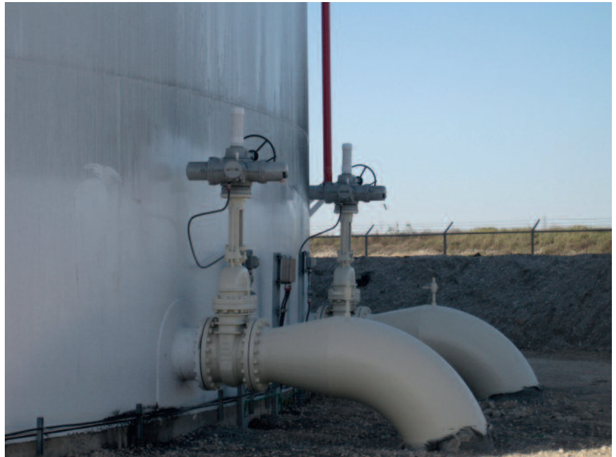
Wireless control technologies are well established in other industries. Here, simplified site wiring and the small antenna on each actuator provide connectivity with the wireless control network
