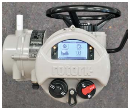
Fig 3 – The actuator indication window is the focus of attention for setting operational parameters and displaying valve, actuator and process information in real time directly at the actuator.
