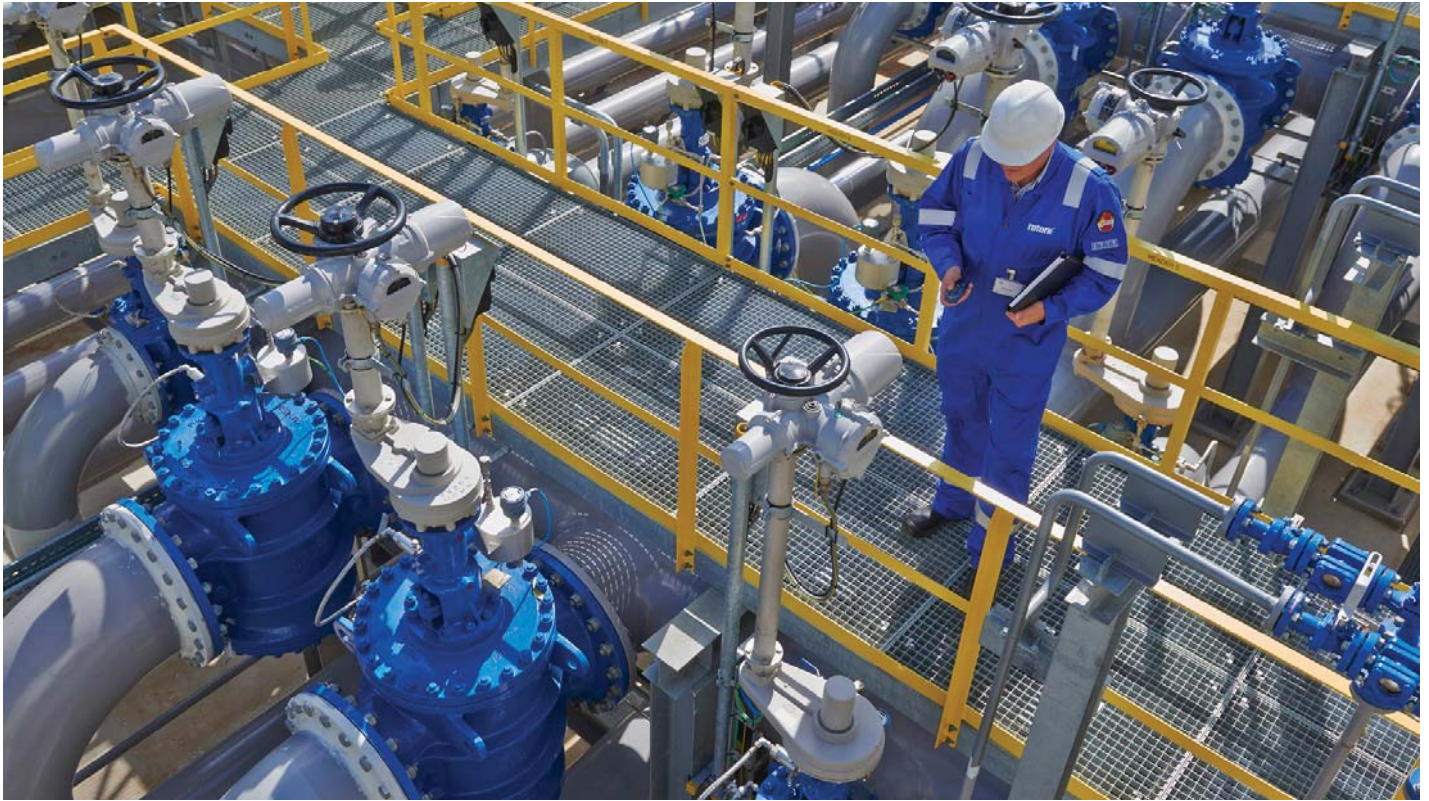
Fig 1 – Because actuators are situated in the critical areas of plant operation, the information that they provide is especially valuable for gauging the health of the process.
