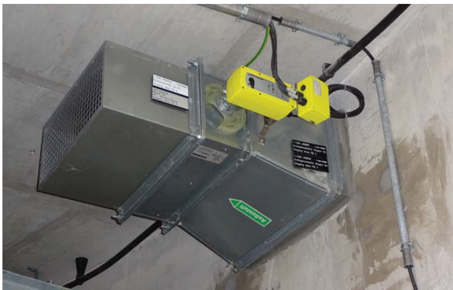
Fig 2: Dampers for smoke and fire protection, as well as air control, are established applications for Schischek actuators.
