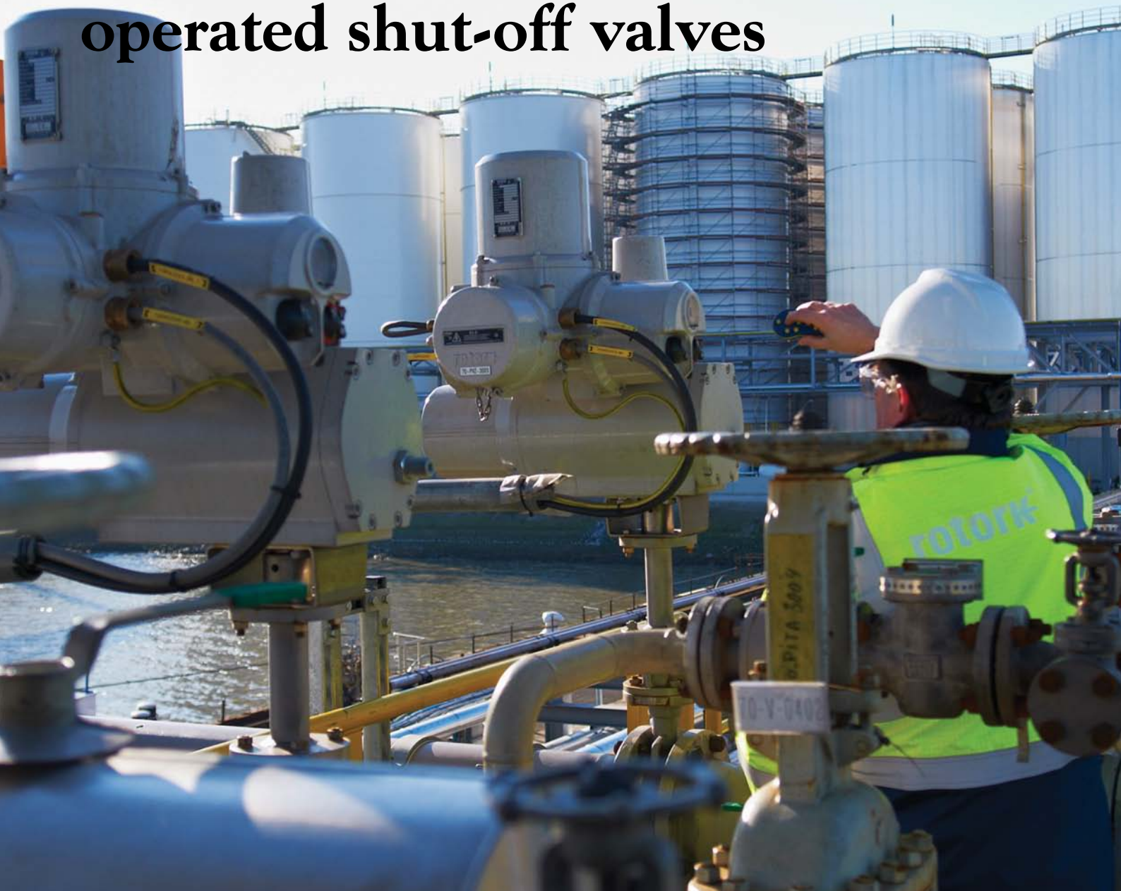
Fig 1 - A Rotork engineer uses the hand-held setting tool that enables non-intrusive programming of Skilmatic actuators and data downloading.
