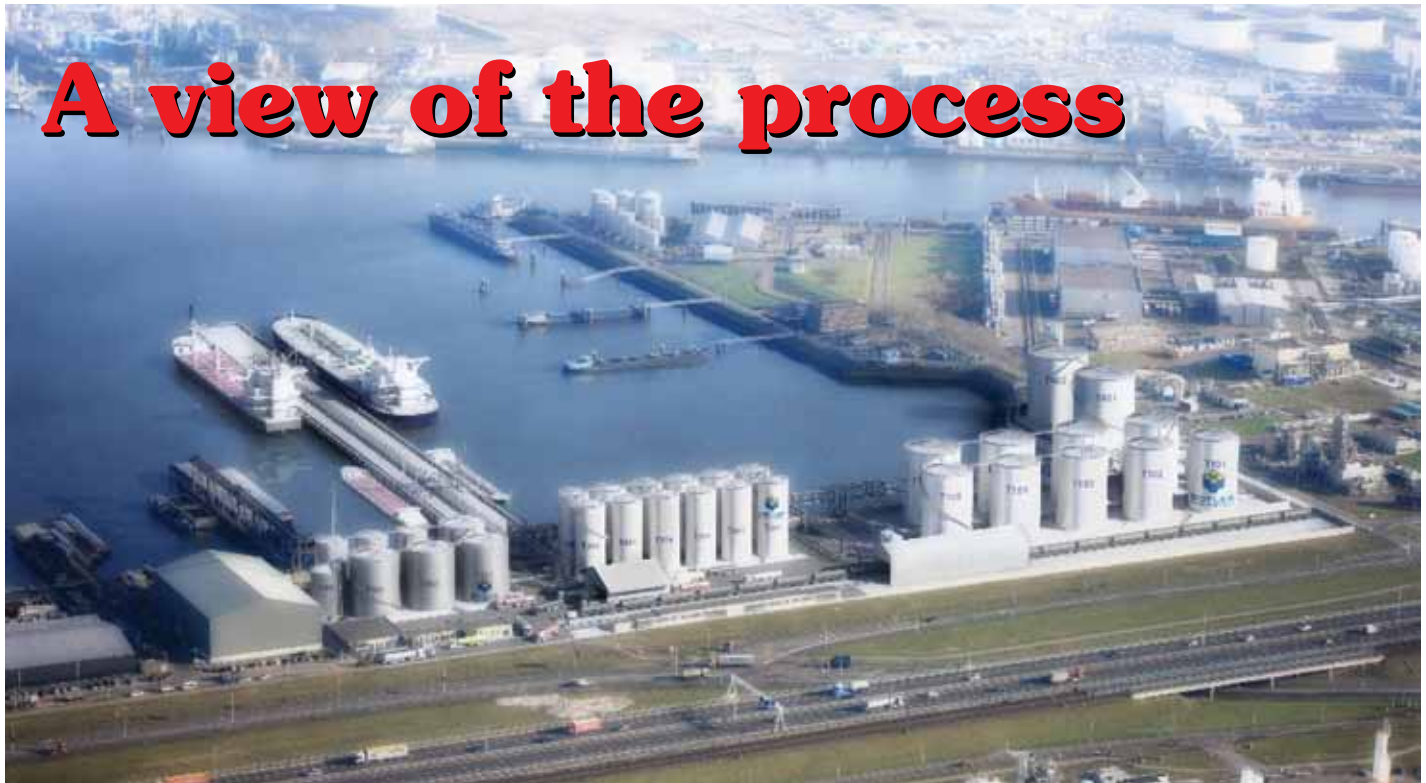
By kind permission from Botlek Tank Terminal B.V.
