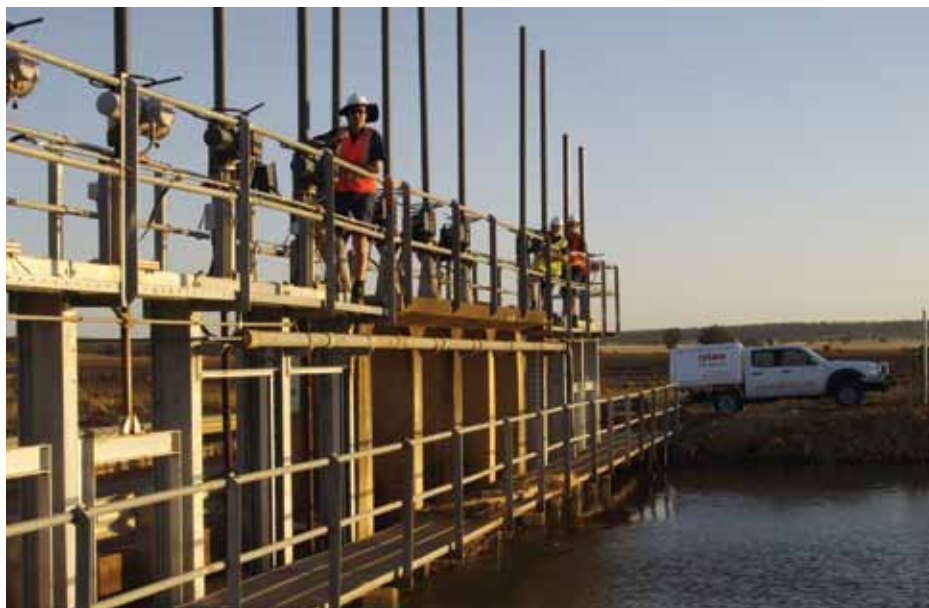
Engineers carry out routine inspection and maintenance at one of the remotely sited river gate installations on the Murrumbidgee Irrigation Scheme.
