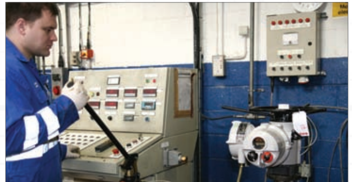
Exeeco's workshop is equipped with custom-built actuator test rigs
