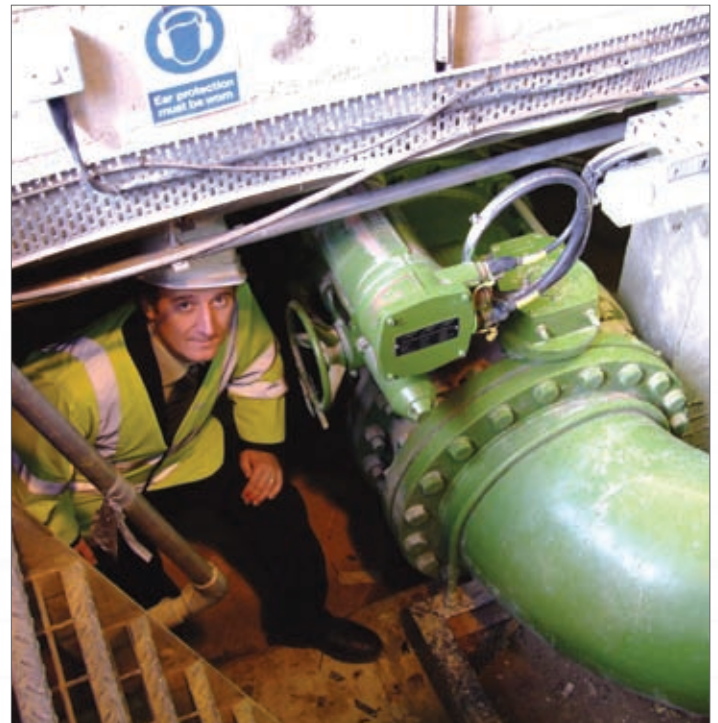
Severn Trent Area Manager Andrew Bowkett with one of the 'A' range actuators in the low lift pump house, which was flooded to a depth of 3 metres
