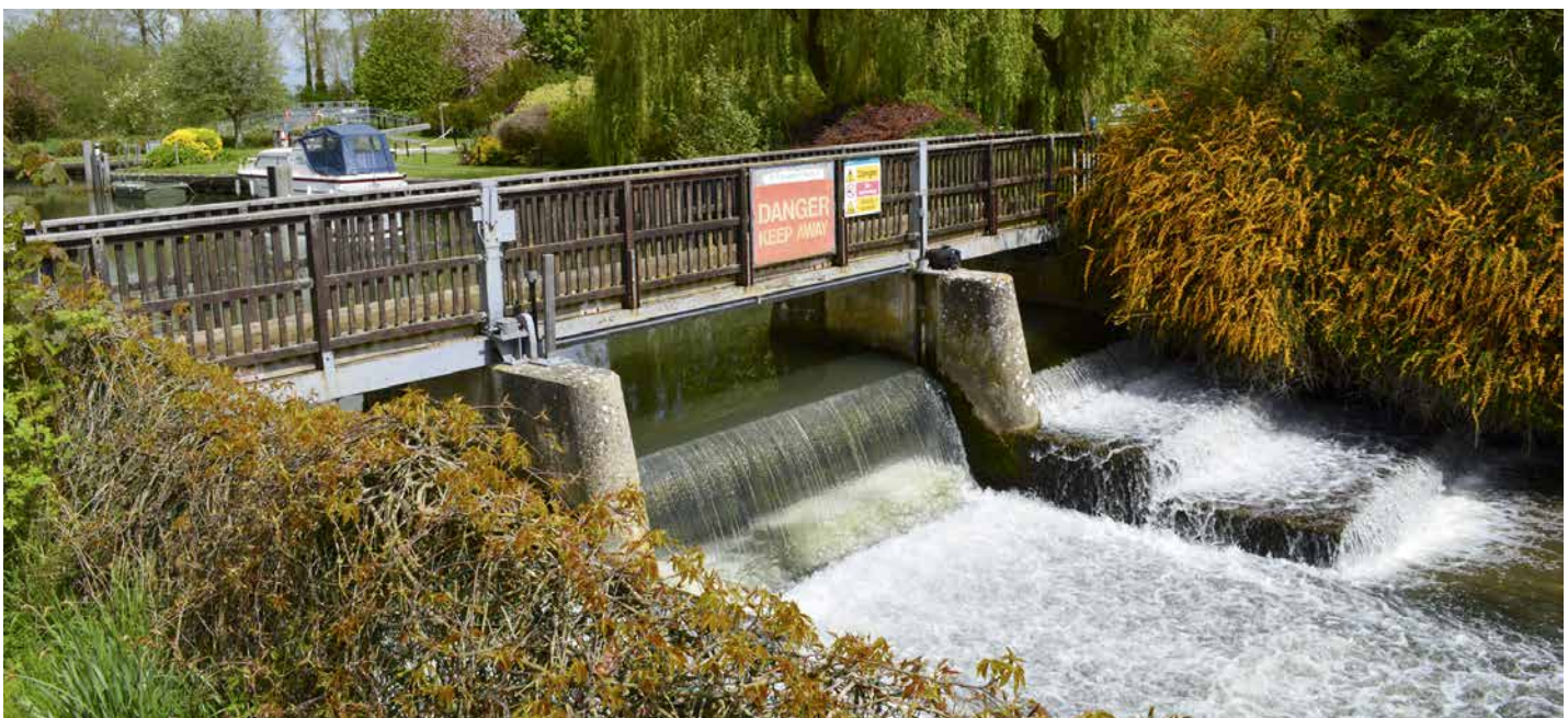
Above: Buscot Weir prior to the upgrade
