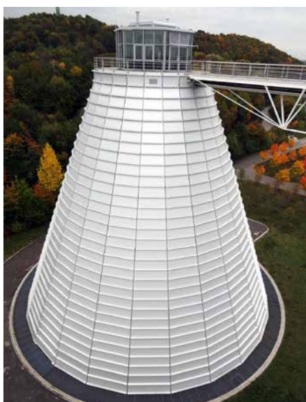
One of the four fermentation tank towers at the Munich waste water treatment works. The Schischek actuators are installed in the lamp at the top of each tower.
