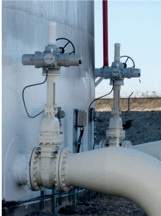
Rotork IQ valve actuator installations on one of the storage tanks at the MMLP Corpus Christi tank farm, illustrating the simplified site wiring (power cabling only) facilitated by the wireless Pakscan P3 control system.
