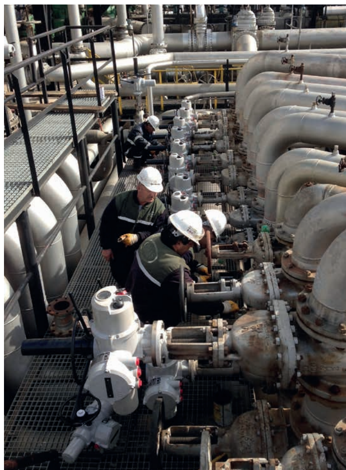
Retrofit work in progress. Engineers from Omas work on one of the tank farm manifolds at the Tupsas Izmit refinery.
