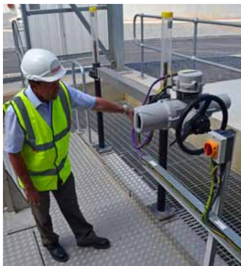
This IQ3 unit, the latest version of Rotork's intelligent actuation product range, drives through Rotork IB gearboxes and extension drive shafts to control the position of the two outlet modulating penstocks on the site's new Ultra-Violet disinfection plant
