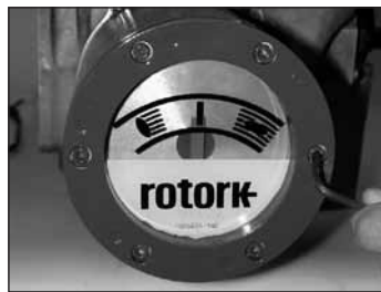
Fig. 8 Valve Position Indicator (Clockwise to Close)
