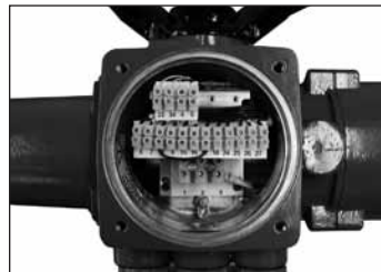
Fig. 7.4 Standard Sealed Terminal Compartment
