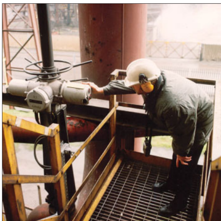
Corus's George Mounsey with the ATEX certified Rotork IQ actuators installed on a 48" gate valve (above) and the Emergency Shut Down (ESD) valve (right) at the Scunthorpe gas booster plant.
