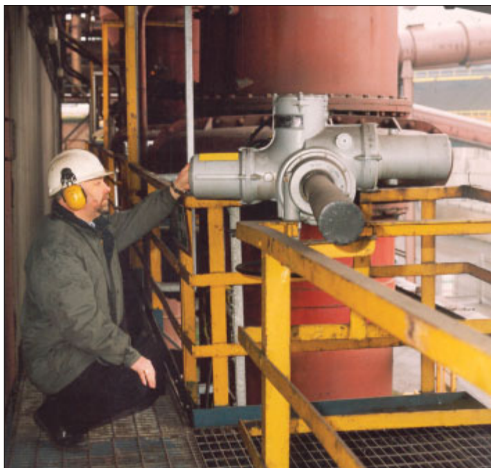
Corus's George Mounsey with the ATEX certified Rotork IQ actuators installed on a 48" gate valve (above) and the Emergency Shut Down (ESD) valve (right) at the Scunthorpe gas booster plant.
