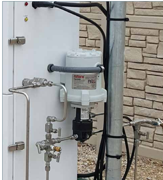
PAX 1 installed on solar powered remote pressure control, station. Low power consumption, Modbus communication and Configurable operating modes enables unmanned control of the distributed Natural Gas Pressure
