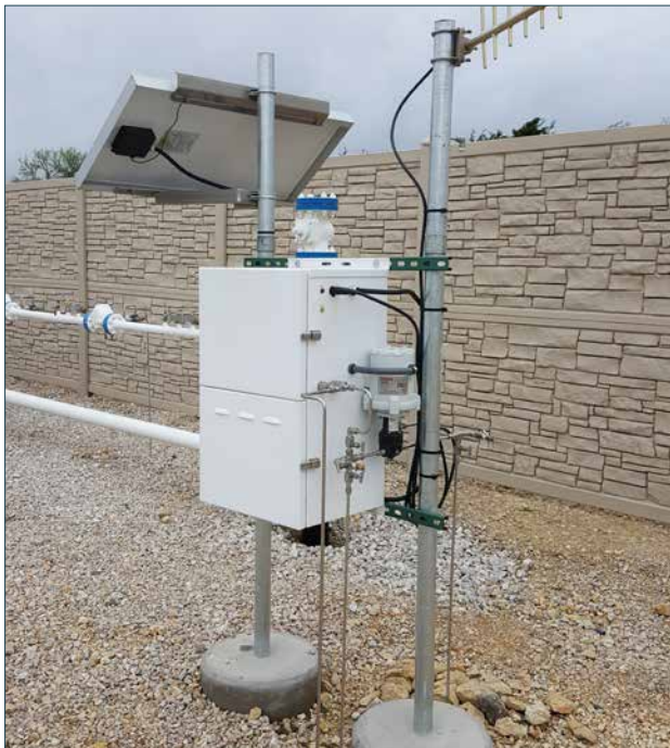
PAX 1 installed on solar powered remote pressure control, station. Low power consumption, Modbus communication and Configurable operating modes enables unmanned control of the distributed Natural Gas Pressure
