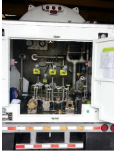
Schischeck ExMax on an LNG transportation tanker
